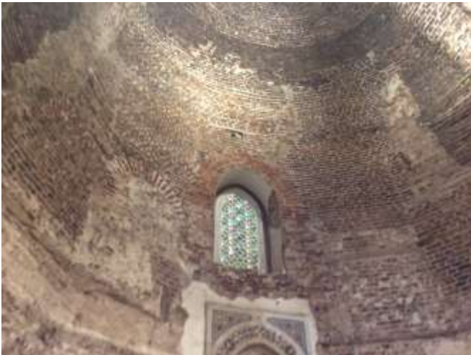
Eastern part of the Church during restoration, 2015
