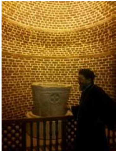
The walls and Baptism after restoration 2015
