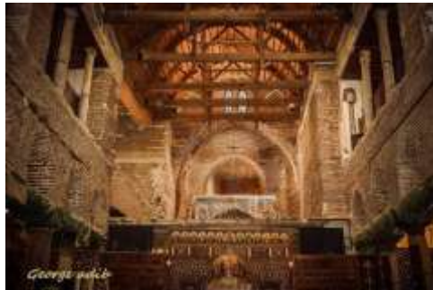
Church during restoration 2015
